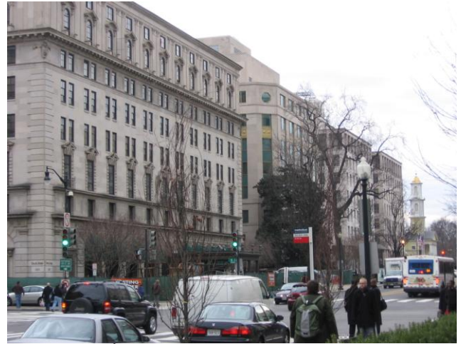
16 th Street opposite project site
