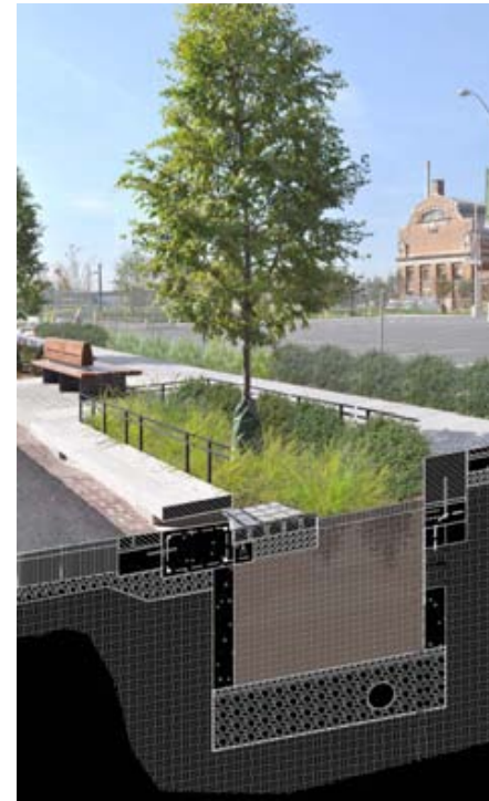
Example of curbside bioretention facility at the Yards, Washington DC
