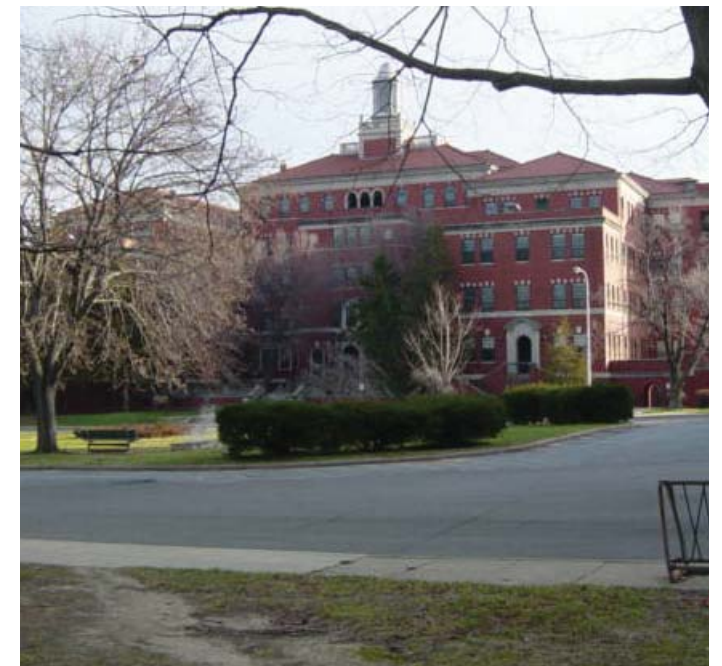
Top: CT Buildings
