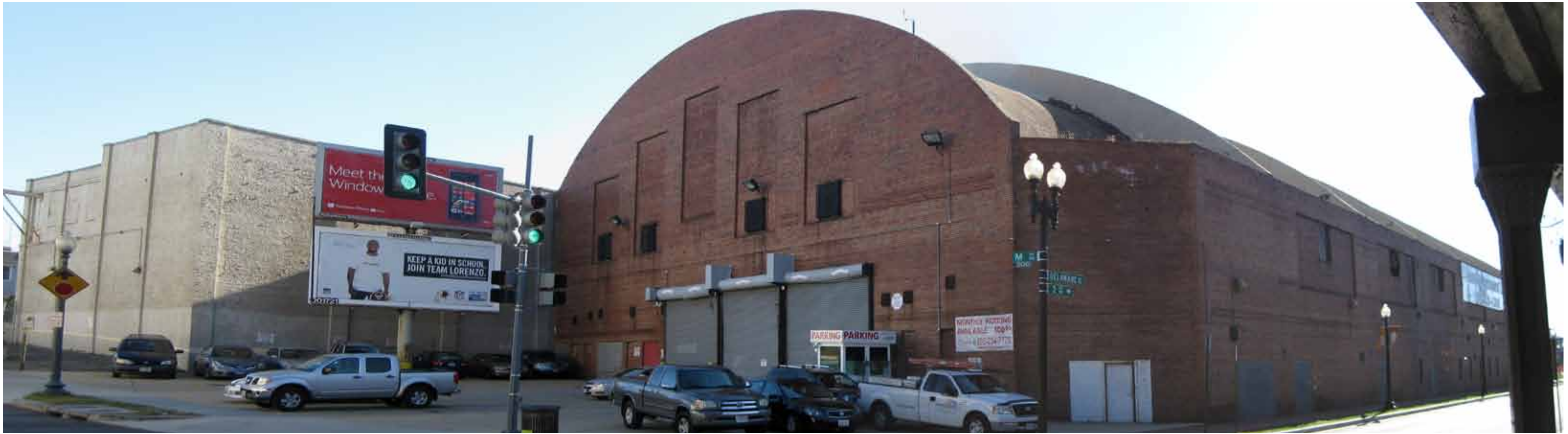
NORTHWEST CORNER WALKING FROM METRO ORIGINAL BUILDING 1941
