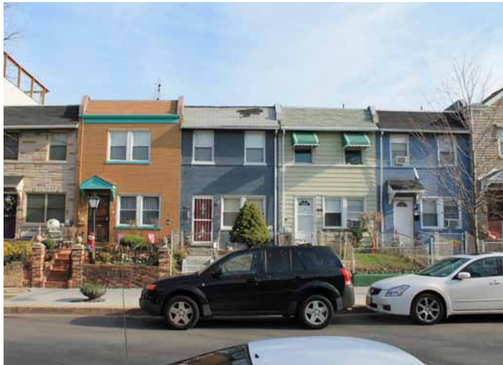
RESIDENCES EAST OF 3RD STREET
