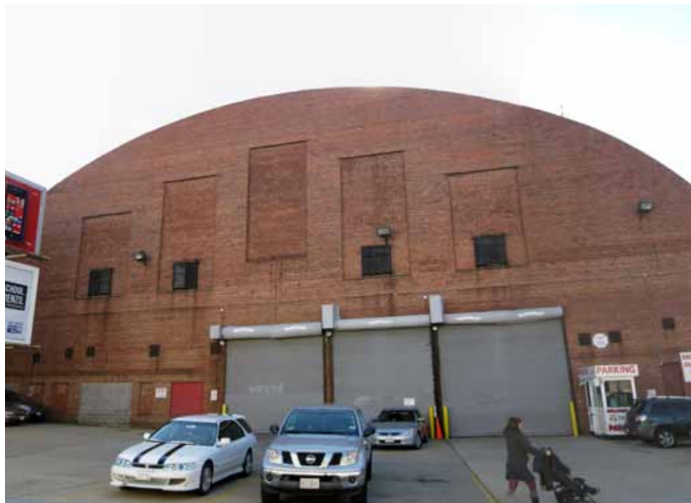
NORTH FACADE FROM M STREET NE
