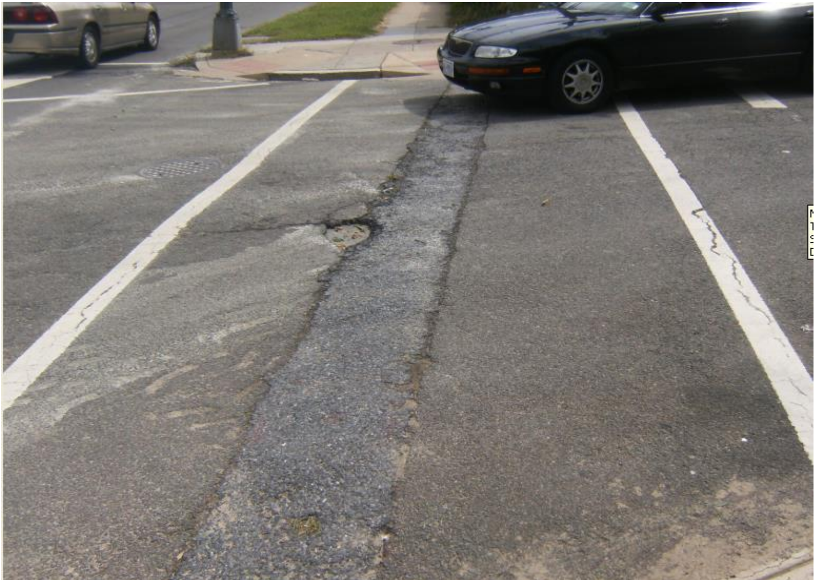
Figure 13. Crosswalk on 2 nd Street (pavement conditions), NW.
