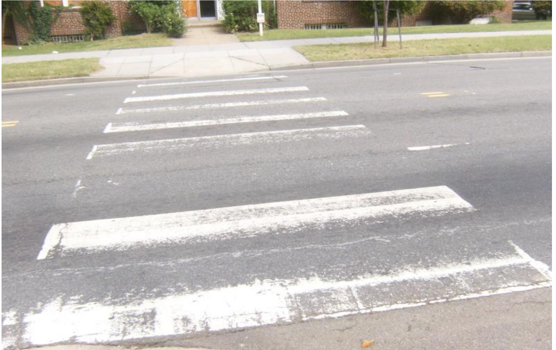
Figure 12. Crosswalk pavement marking on Missouri Avenue close to Jefferson Street, NW.
