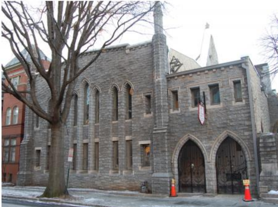
Cloisters served as a transition in scales from the parish hall to the larger church at the end.
