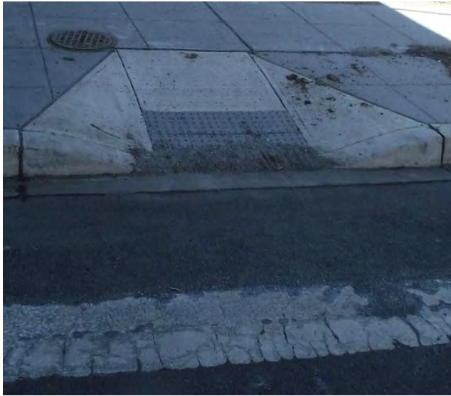
Figure 14 – Non-Standard Pedestrian Ramp
