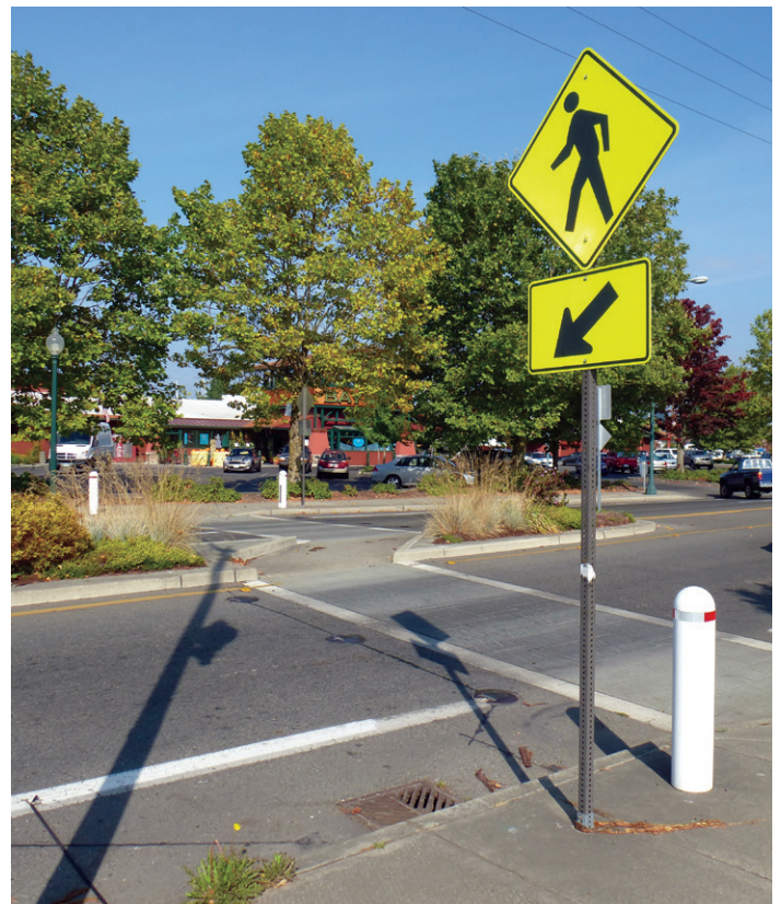
Raised Median with Pedestrian Safety Island
