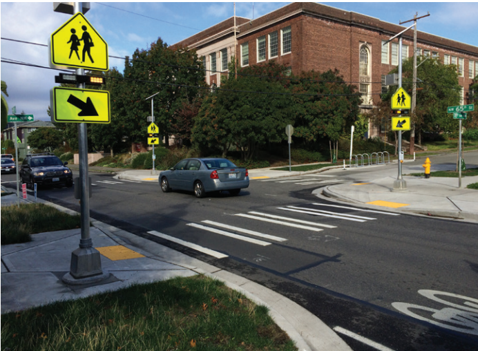
Rectangular Rapid Flashing Beacons (RRFB)
