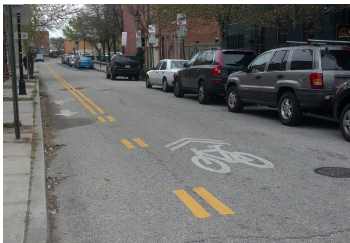
Counterflow Bike Lane on Lancaster Street
