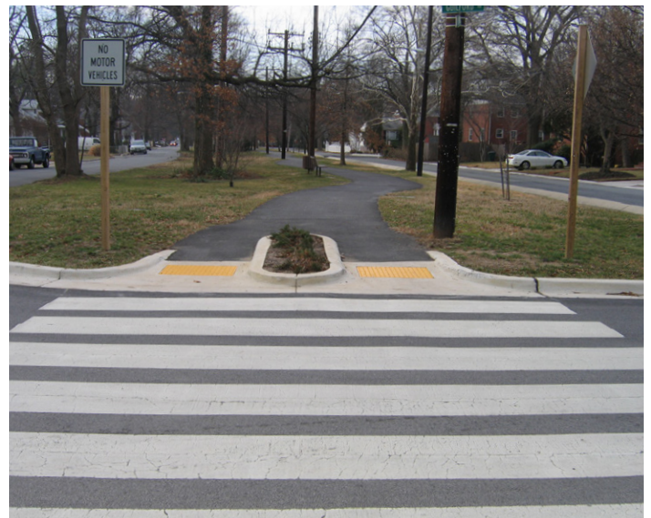
Sidewalk Ramp on a Shared-Use-Path in College Park, MD
