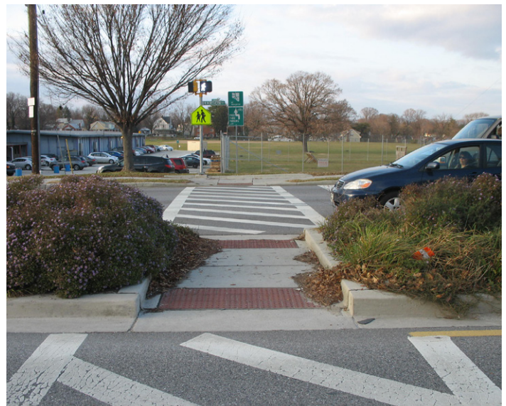
Pedestrian Safety Island on Northern Parkway
