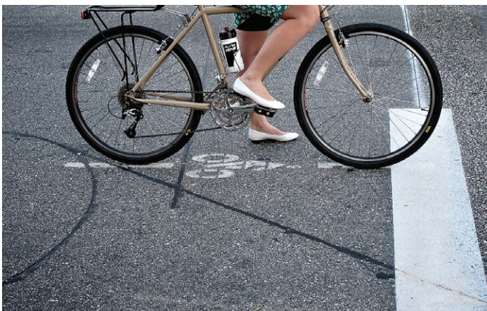
Pavement Markings Indicate the Bicycle Signal Detection Location
