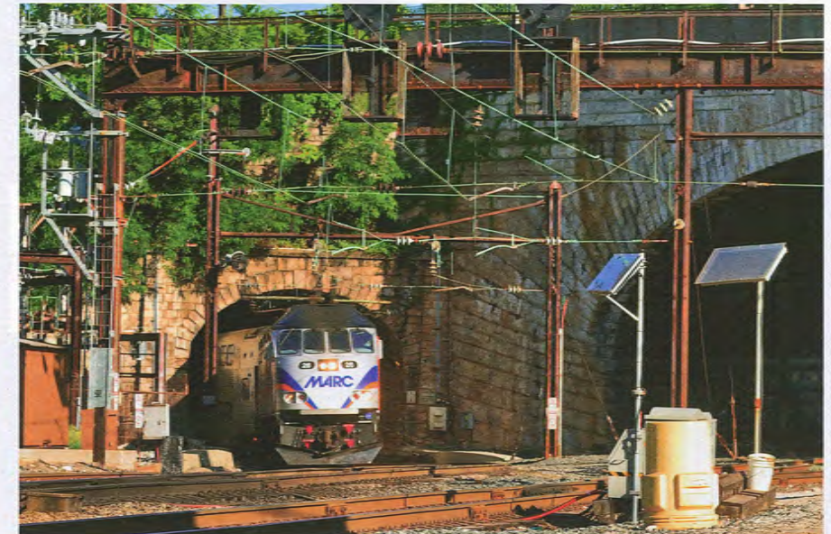
A MARC train exits the tunnel shortly before its arrival at Baltimore Penn Station. While MARC would be a major beneficiary of the new tunnel, it has no role in the project. Mitch Goldman
