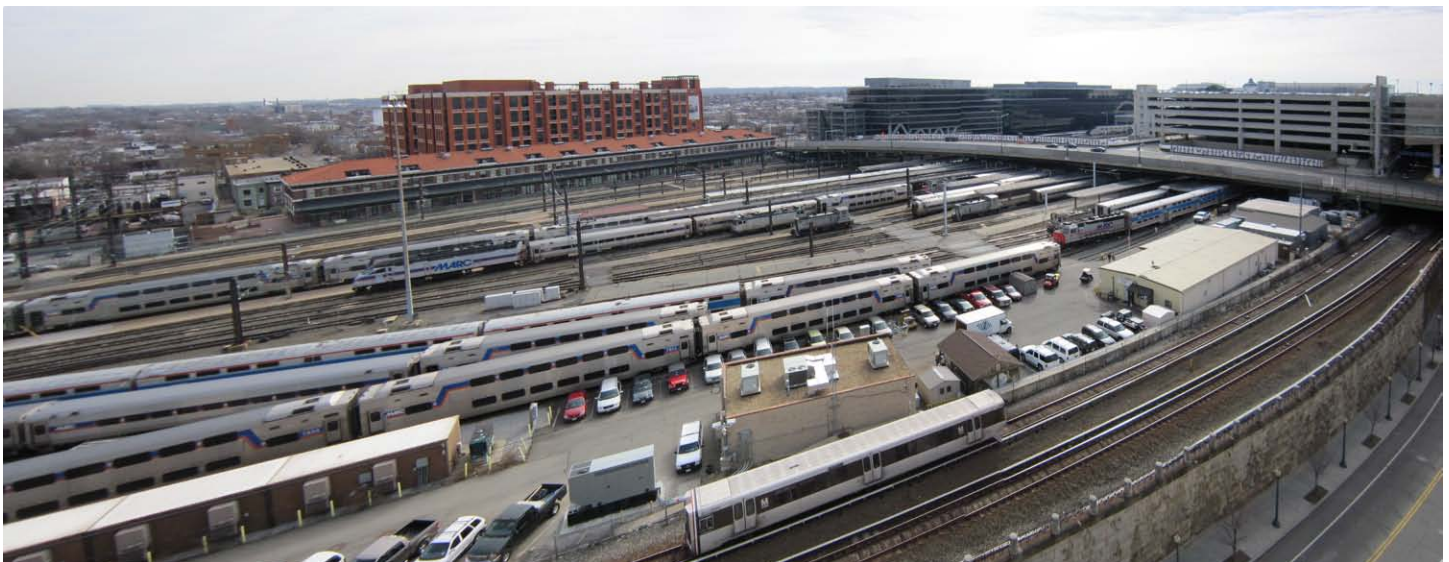
View of station looking southeast showing midday storage of equipment on active platforms
